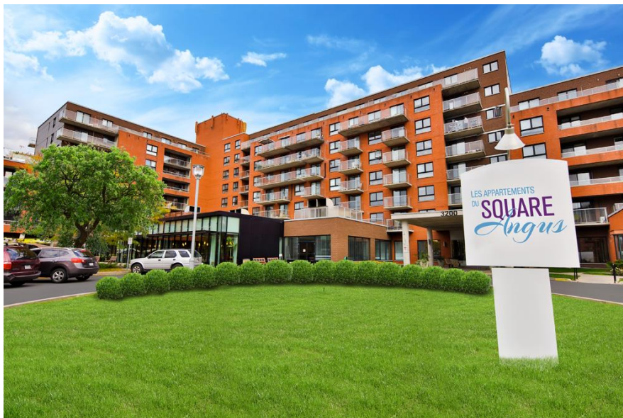
Figure 1- Les appartements Square Angus (2015)
