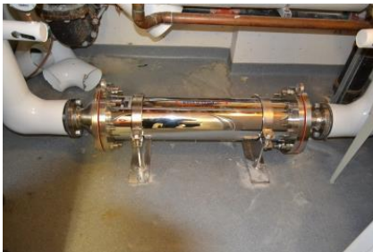
Figure 5: Mag-O-Pure Catalyzer with an Anti-Lime Treatment Capacity of up to 300 gpm
