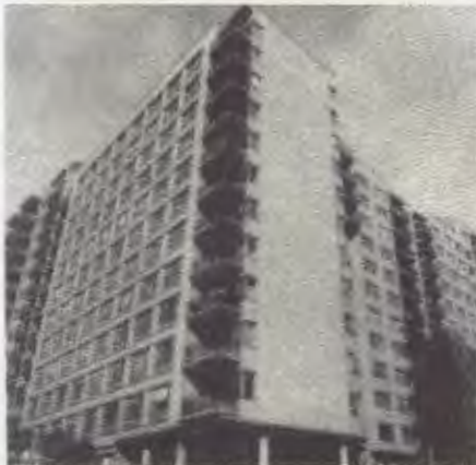
At Mountain Place Towers, a large Montreal apartment complex, building management was faced with problems of maintaining proper comfort levels with existing HVAC equipment.
